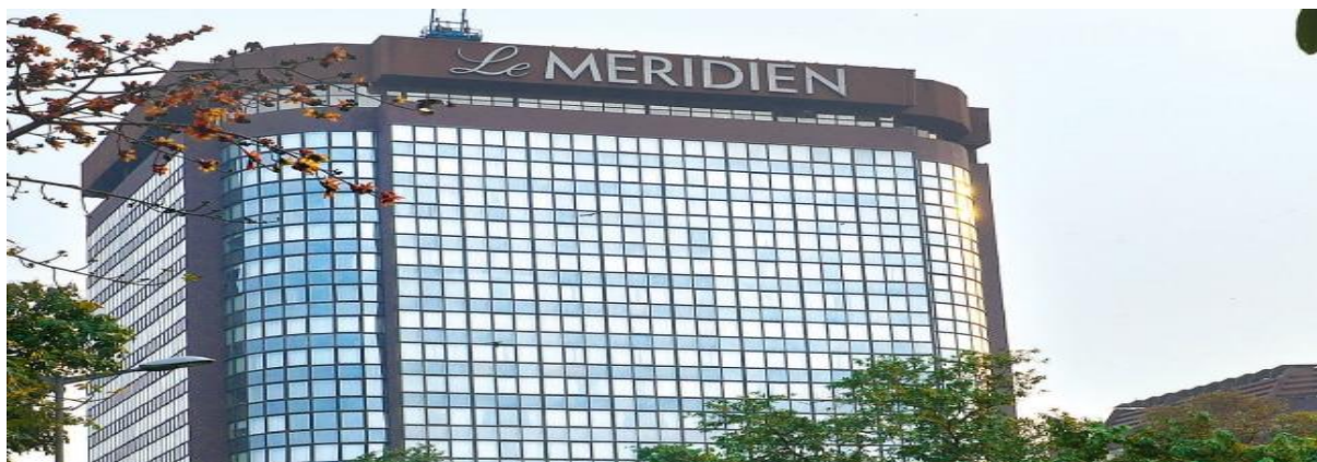
Figure 1.3-2 First Glass curtain wall Building in India
