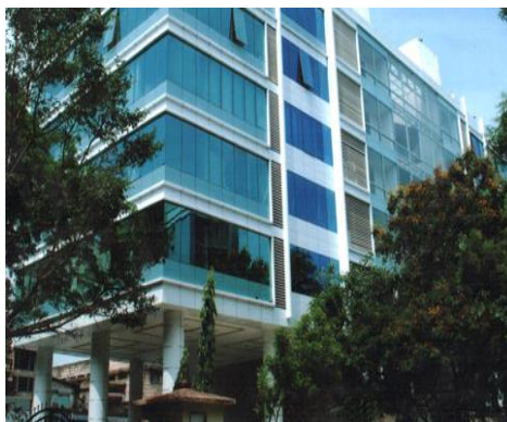
Figure 3.1-4 Building on Stilts (Mumbai)
