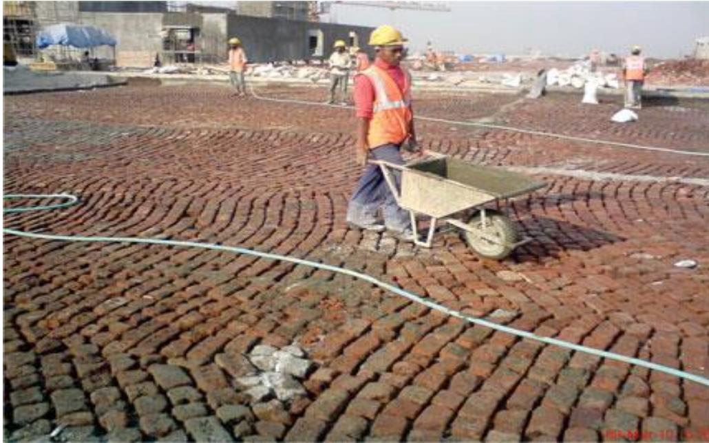
Figure 3.3-2 Brick coba ovr RCC slab in Mumbai
